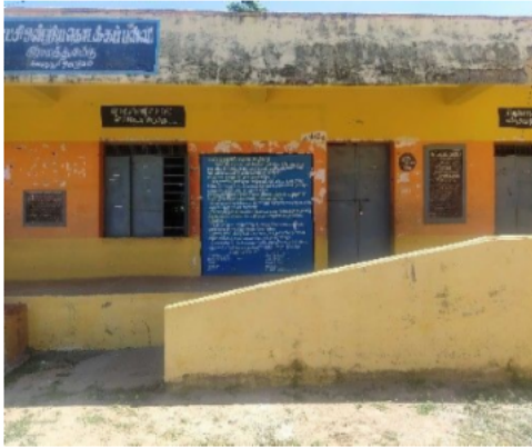
Polling Station Building Front View
