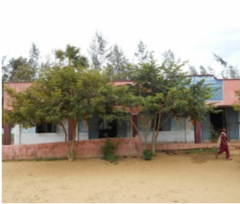
Polling Station Building Front View
