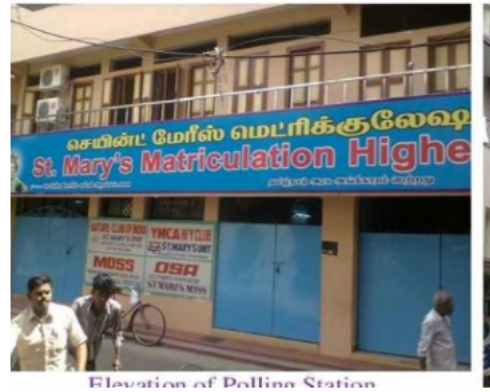
Elevation of Polling Station
