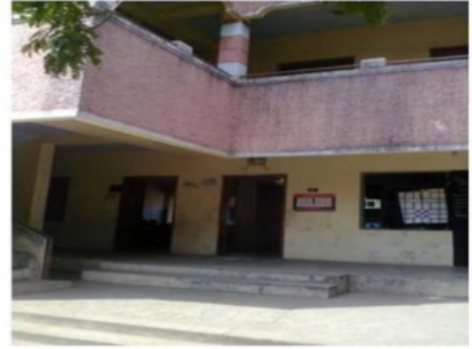
Elevation of Polling Station
