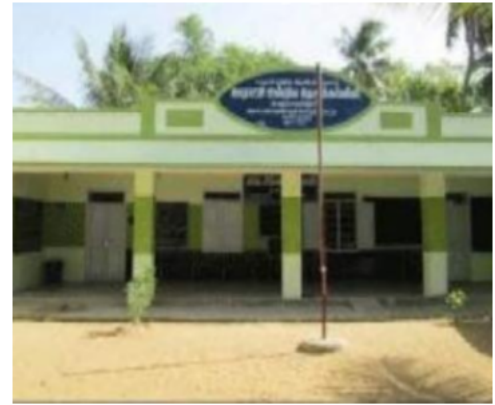
Polling Station Front View
