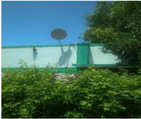
Polling Station Building Front View
