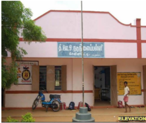
Polling Station Building Front View
