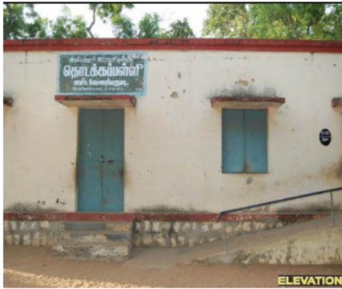
Polling Station Building Front View
