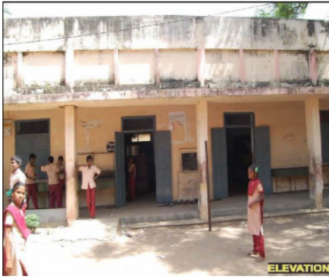
Polling Station Building Front View
