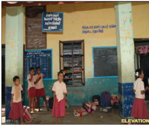
Polling Station Building Front View
