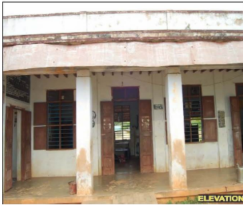
Polling Station Building Front View
