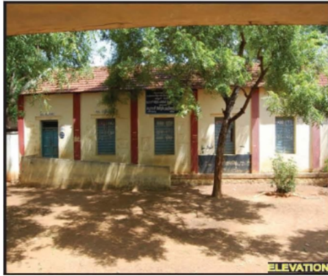
Polling Station Building Front View
