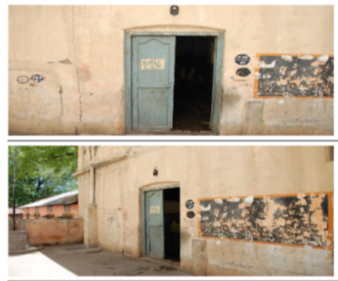
Polling Station Front View
