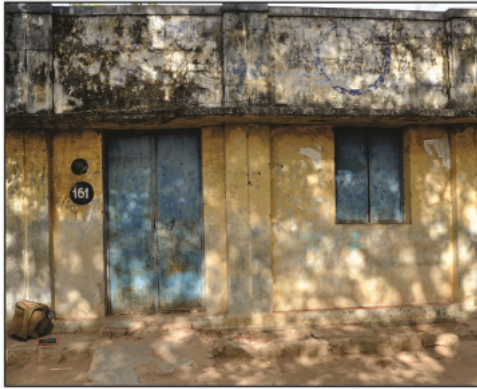
Polling Station Building Front View
