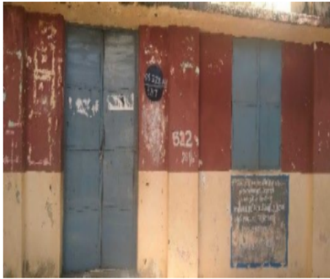
Polling Station Building Front View
