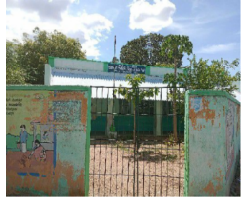
Polling Station Front View
