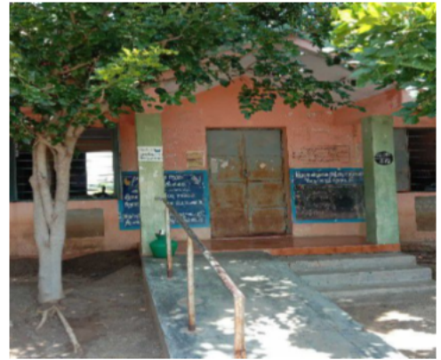
Polling Station Front View
