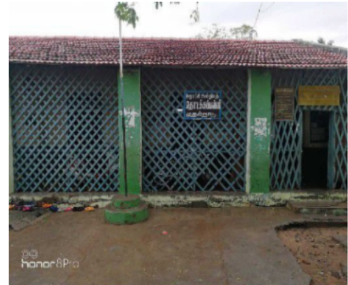
Polling Station Front View
