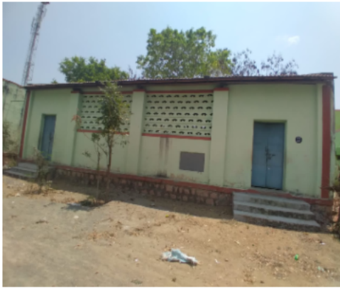
Polling Station Building Front View
