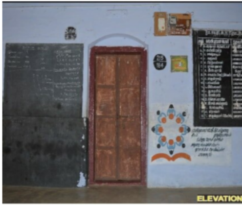
Polling Station Building Front View
