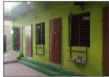
Polling Station Front View
