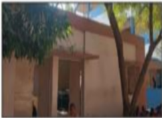
Polling Station Building Front View
