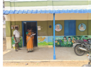
196-Panchayat Union Primary School, Southern portion-Sevalkulam
