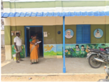
196-Panchayat Union Primary School, Southern portion-Sevalkulam
