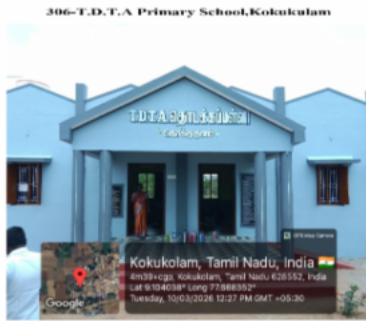
Polling Station Building Front View
