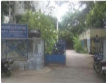
Polling Station Building Front View
