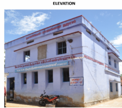
Polling Station Front View
