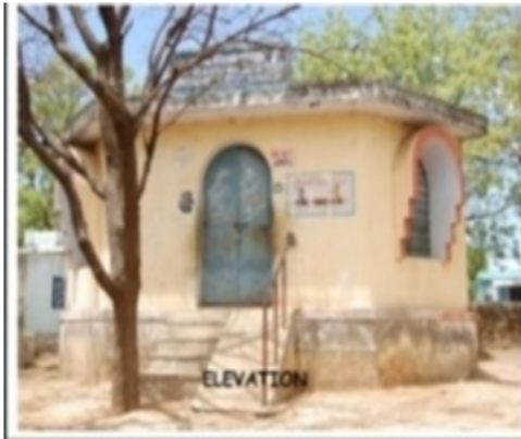
Polling Station Building Front View
