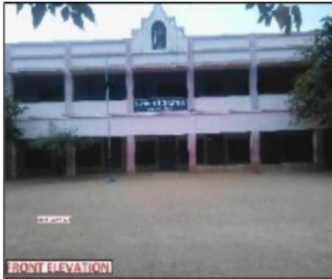
Polling Station Building Front View
