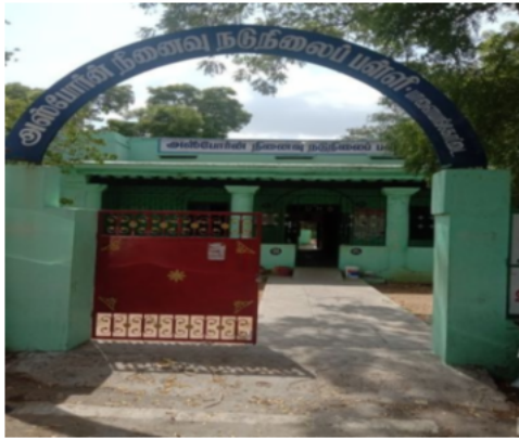
Polling Station Building Front View
