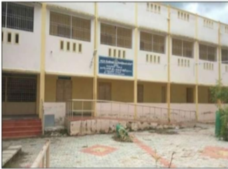
POLLING STATION FRONT VIEW
