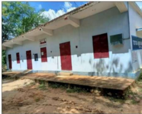
POLLING STATION FRONT VIEW
