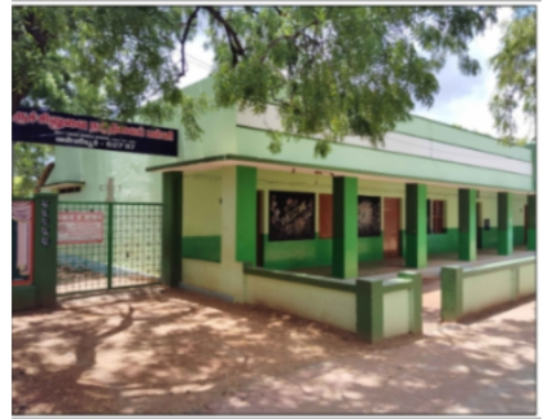
POLLING STATION FRONT VIEW
