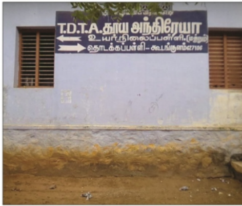
Polling Station Building Front View
