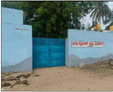
POLLING STATION FRONT VIEW
