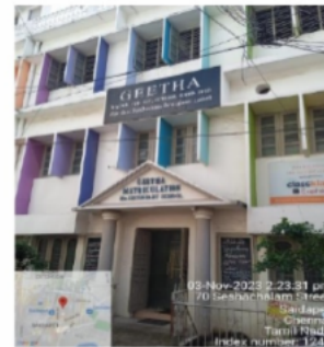
Polling Station Building Front View
