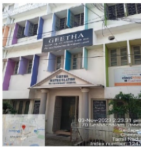
Polling Station Building Front View
