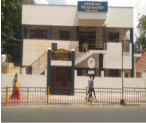
Polling Station Building Front View
