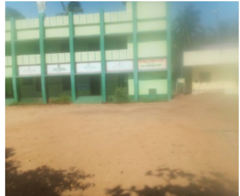
Polling Station Front View
