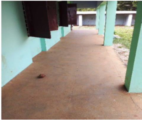
Polling Station Building Front View
