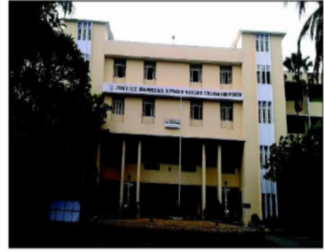
ACTUAL PHOTOGRAPH OF POLLING STATION
