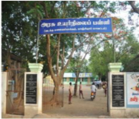
Polling Station Building Front View
