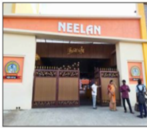
POLLING STATION BUILDING FRONT VIEW
