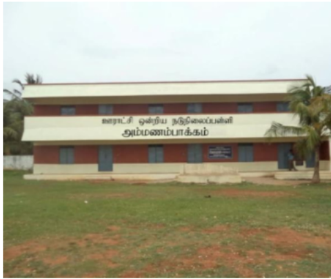
Polling Station Building Front View
