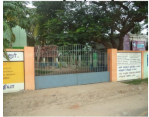
(3) ACTUAL PHOTOGRAPHY POLLING STATION.
