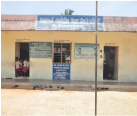
Polling Station Building Front View
