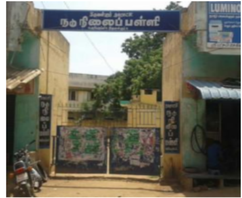
Polling Station Front View
