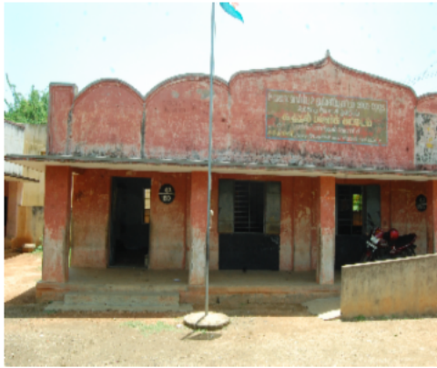
Polling Station Building Front View
