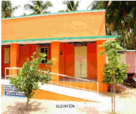
Polling Station Building Front View
