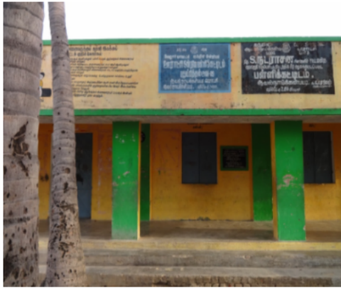
Polling Station Building Front View
