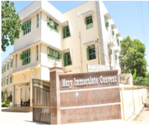
Polling Station Building Front View
