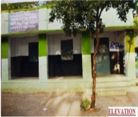
Polling Station Building Front View
